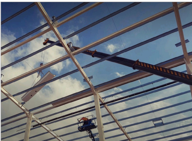
Gutters being craned through the purlins with next purlin up from the gutter being left out for access
