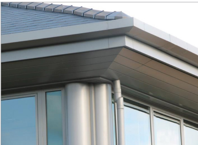
Figure 2: Eaves gutter enclosed by fascia/soffit
