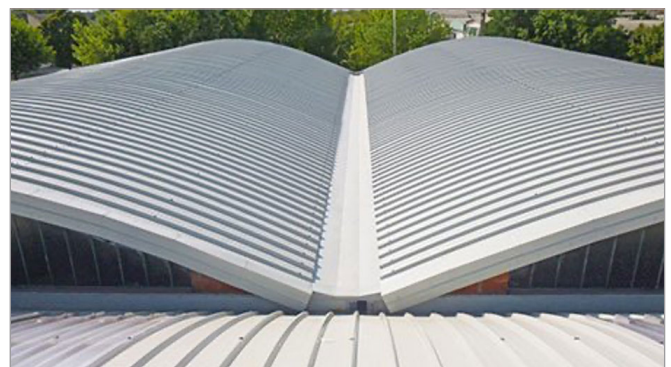
Figure 3: Insulated membrane lined valley gutter
