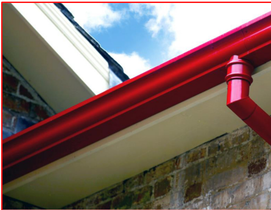
Figure 1: Typical external eaves gutter
