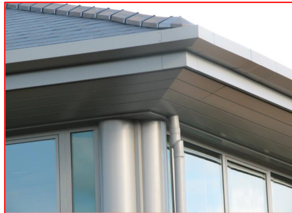
Figure 2: Eaves gutter enclosed by fascia/soffit
