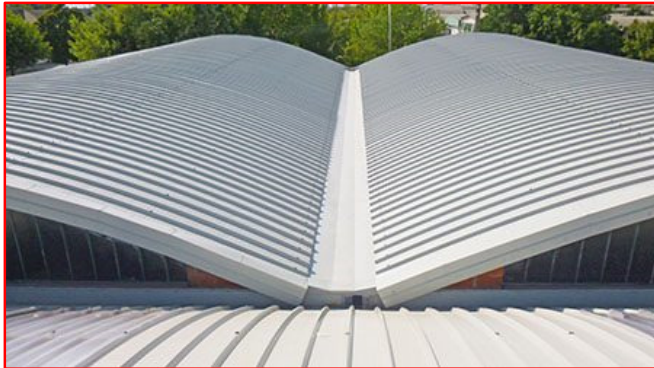
Figure 3: Insulated membrane lined valley gutter
