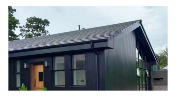
Marley Alutec's Evolve Deepflow, Tudor downpipes and Evoke fascia and soffit products have been selected for a new self-build residential property in Lanarkshire. The aluminium rainwater and roofline systems were chosen for their durability, high quality appearance and ease of installation, as they were fitted by the homeowners themselves.
