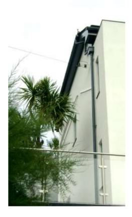
Sleek and unobtrusive, Alutec's Evolve aluminium gutter range comes with a unique patented Jurajoint system for quick, simple and secure jointing – as easy as PVC. The Deepflow profile has a flow rate of 4.9 l/s and 232m² per downpipe making it ideal for the coastal weather conditions of the project. Furthermore, with a lead time of only two days on Heritage Black and Anthracite Grey products, Andy and his team received the system quickly and could begin installation as soon as possible.
