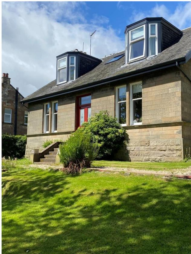
A combination of products from Marley Alutec have been used on a Victorian residential property near Glasgow. The company's Evolve Half Round and Traditional Moulded Ogee aluminium rainwater systems were selected as a durable and low maintenance like-for-like replacement for traditional cast iron.
