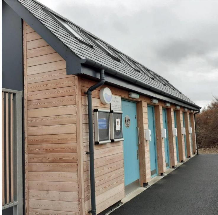
The new facility at Longniddry Bents Car Park features Marley Alutec's Evoke fascia and soffits, as well as its Evolve half round gutter and 63mm downpipe all in a uniform RAL7016 anthracite grey. By specifying Marley Alutec's marine-grade and composite aluminium material, the new build's guttering system has a functional life expectancy of 50 years with minimal maintenance needed over that time.
