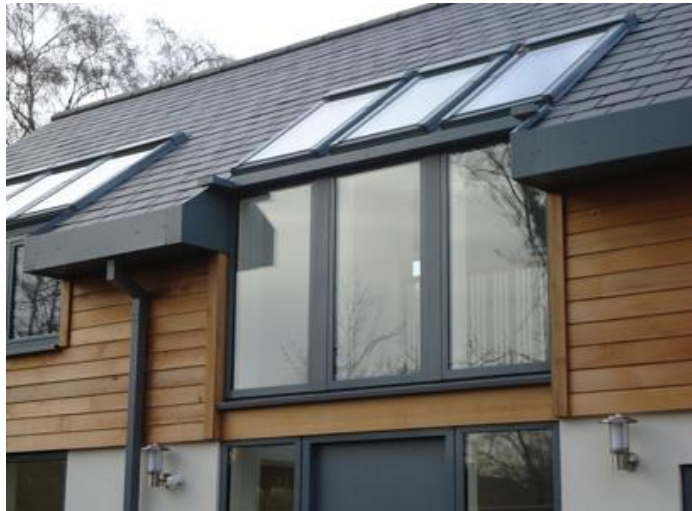
Example of a well-maintained gutter system
