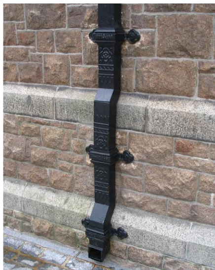
A cast iron drainpipe at Guernsey Market, St Peter Port, Guernsey
