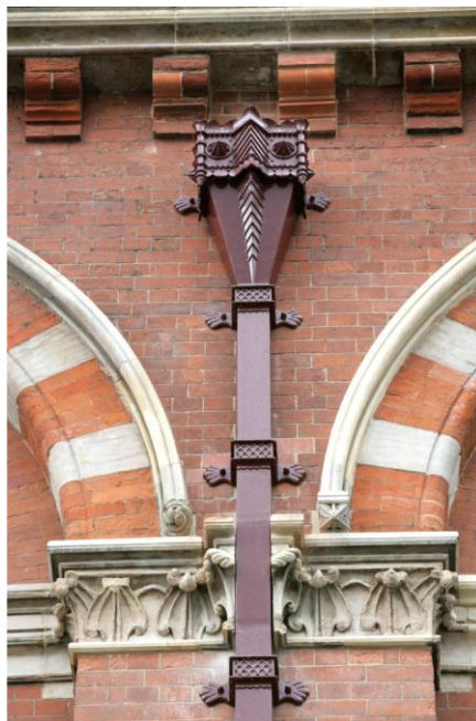
A cast iron hopper at St Pancras International Station, London
