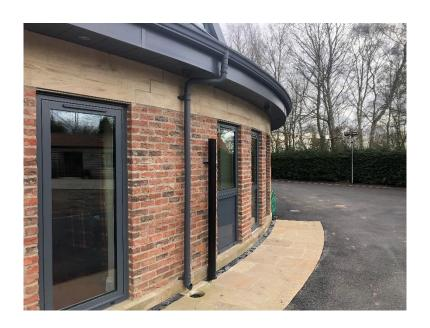
Metal roofline product specialist ARP has manufactured bespoke version of its Legacy heritage-style cast aluminium guttering for a unique house in Yorkshire. Oaklands, built by Cohesion Construction, is a completely round house with an interior core which features an outdoor dining area and fire pit. The house's unique design presented ARP with a challenge to produce guttering for both the internal and external curved roofline.
