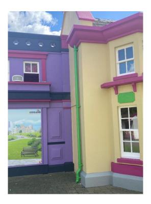
Choosing aluminium for the guttering was the logical choice for Legoland. As well as the colour options available, aluminium is maintenance-free and will retain its striking good looks even in a tough environment like a theme park. Incredibly hardwearing, resistant to the elements and corrosion, cast aluminium can be used to create rainwater systems to suit any style of architecture.
