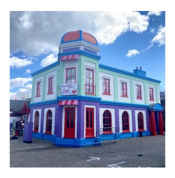
A major refurbishment project at Legoland near Windsor has certainly tested ARP's boast to produce aluminium guttering, downpipes and fittings in any colour to the limits! Shocking pink guttering, bright red hoppers and bright blue downpipes to match Lego's official colours all feature on buildings across the Berkshire site that were refurbished during lockdown.
