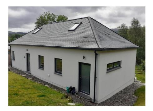
Unusually, the Evoke material supplied to the project did not include any pre-cut, pre-formed or bespoke elements. Instead, standard sheets of the composite aluminium panel were delivered to site and the contractor team cut and formed each section to fit the shape of the building.
