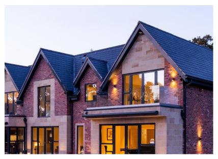
Evoke fascia type A was used on the sloping eaves and type B on the bargeboards. Bespoke box end corners were designed to ensure the transition from eaves to bargeboard was unobtrusive yet easy to install. Evolve Ogee rainwater goods and Flushfit pipes were chosen to complement the contemporary nature of the build, all in RAL7016 anthracite grey.
