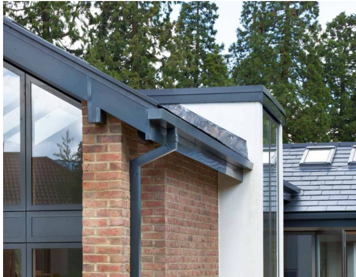
Box gutter and 72x72mm downpipe in RAL 7021 granite grey
