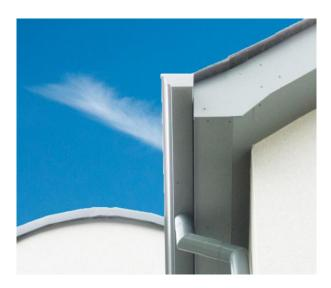
Aluminium fixing brackets are clipped into position at centres not exceeding 450mm as roll forming is continued. The formed gutter is cut to length and a stop end fitted to the remaining open end.
