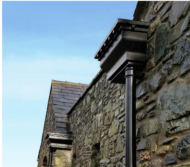
Hoppers and downpipe
