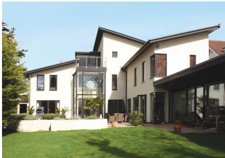
Aluminium soffit, fascia, downpipe, box gutter and capping
