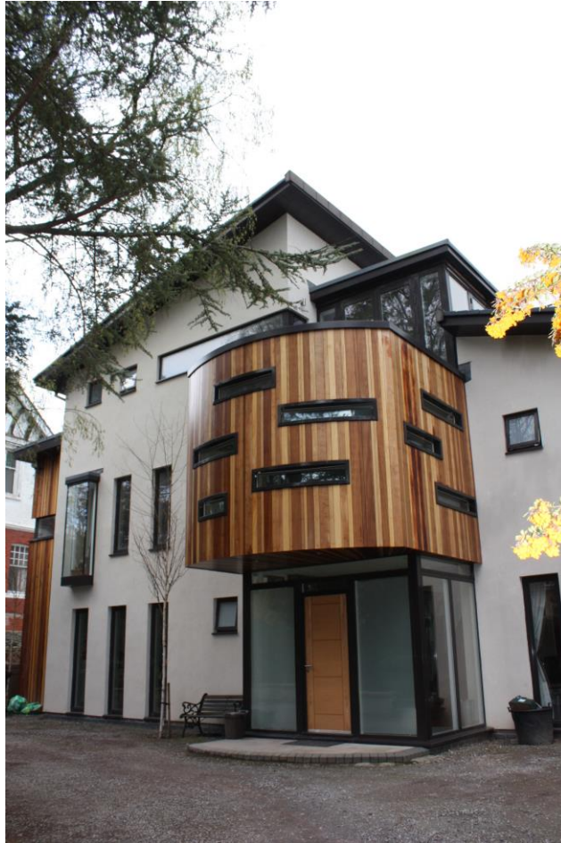
Aluminium capping, soffit and guttering
