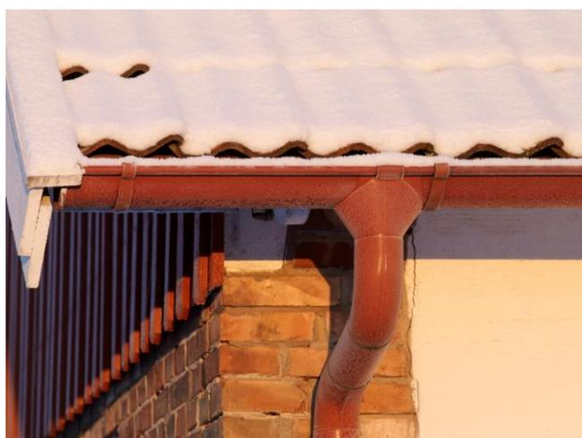
The correct position and height of the gutter needs to be carefully determined, for example, whilst a lower level fitted gutter is less susceptible to sliding snow, it could result in wind driven rainwater going between the back of the gutter/roofline which can lead to water damage to the building fabric. A gutter fitted at a higher level will alleviate this problem.
