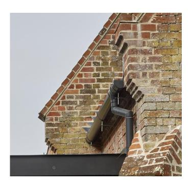
Also specified for the build was Alutec's Evolve Deepflow rainwater system, including the Flushfit downpipe in 76mm. Ideal for larger properties such as this 340 square metres home, the system has a flow rate of up to 4.9 l/s and 232m2 per downpipe. Manufactured from marine grade aluminium, it is highly corrosion resistant and will never need re-painting.
