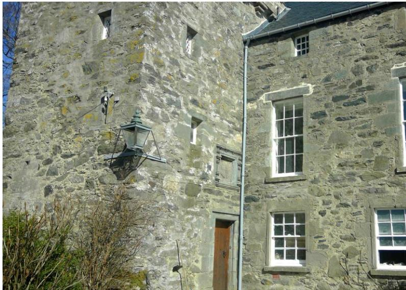
Archie specified Legacy cast aluminium deep flow guttering, as it is made from cast aluminium and is specifically designed to replicate cast iron. However, in this instance, allowance was made for a higher flow capacity for the rain and melted snow. The gutters were teamed with Colonnade cast collared rainwater downpipes, which again mimics the look of cast iron to provide the heritage style required to suit the property.
