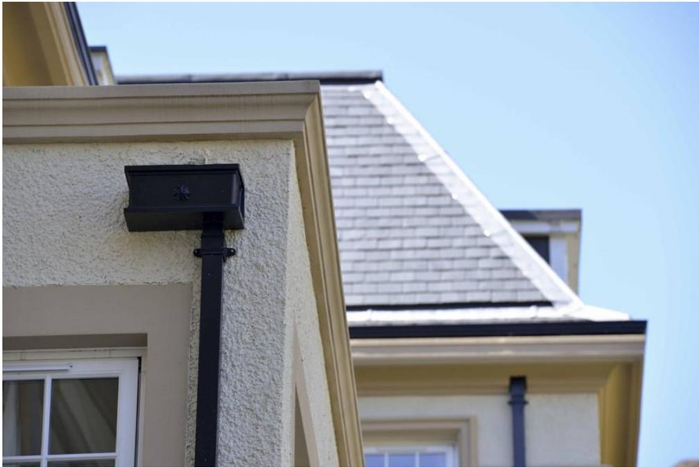
The architects specified the Aligator Ogee No. 46 gutter with Traditional 102mm x 76mm downpipes. Alutec’s Aligator Snapfit gutter jointing system features an internal ‘Snap-fit’ union and a concealed fascia bracket to provide a smooth, uninterrupted line at the eaves of a building – perfect for a project like Ardgartan Hotel where there is a classic design requirement.
