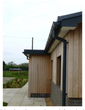
Colonnade swaged aluminium downpipes are also made from aluminium and are perfectly compatible with the Sentinel gutter system. Working together they provide a high quality, low maintenance rainwater system that will last for more than 30 years.
