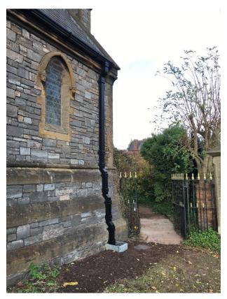
The sizeable order included Britannia cast iron moulded ogee gutter and rectangular cast collared downpipes. These products were chosen for this project specifically as it is a high quality and conservation equivalent product ensuring that all heritage considerations were adhered to. The profiles and painted finish are in keeping with the traditional style of the building and Britannia cast iron is expected to last for at least 100 years, providing it is maintained and repainted regularly.
