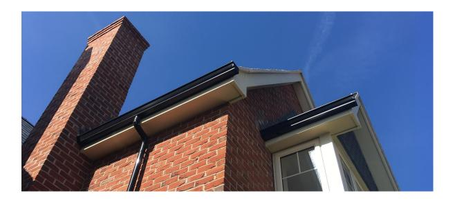
Mustang® Aluminium Seamless Guttering is a unique joint-less system and is the only seamless gutter system approved by the British Board of Agrément (BBA). ARP recently celebrated their 25th year of continuous certification and in meeting the strict BBA guidelines, both ARP and their approved installer network are audited and assessed twice yearly to ensure that the product and installers maintain these high standards.
