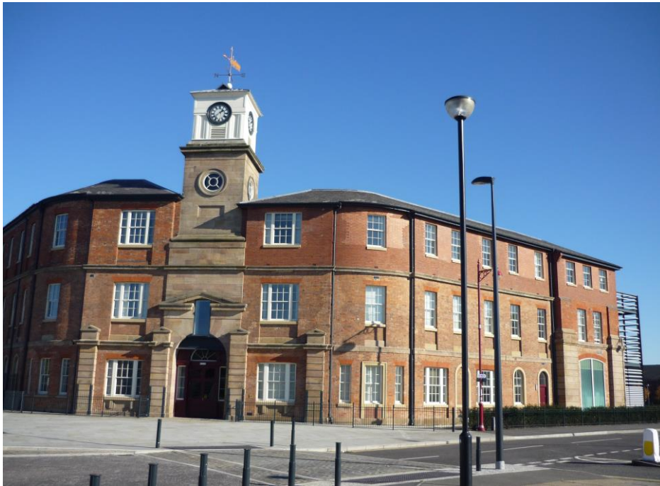
The Grade II listed Roundhouse Building, Derby Image courtesy of Saint-Gobain PAM UK
