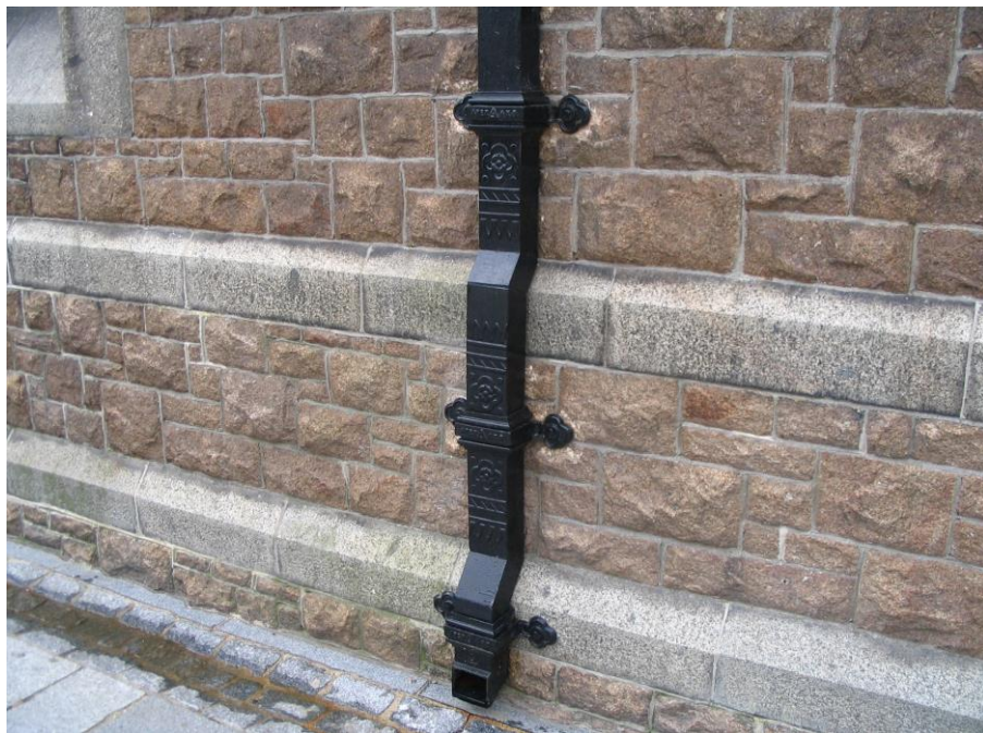
Cast iron downpipe installed at Guernsey Market, St Peter Port Image courtesy of Alumasc
