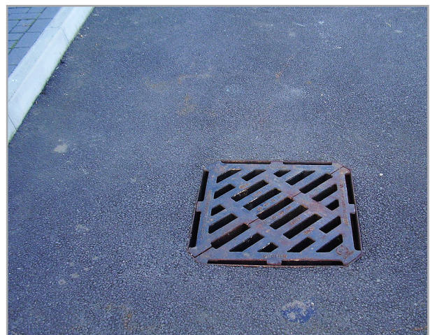
Vented lid on discharge manhole
