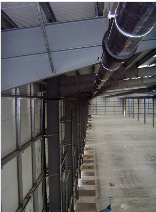
Siphonic pipework horizontal at high level
