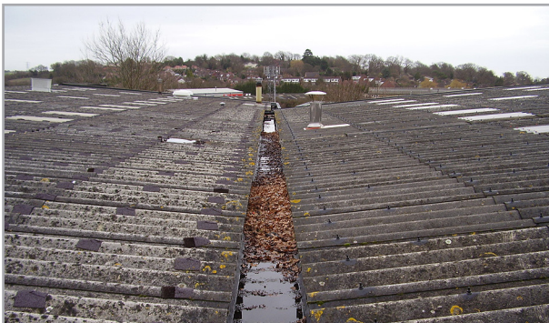
Even good designs will fail if not maintained
