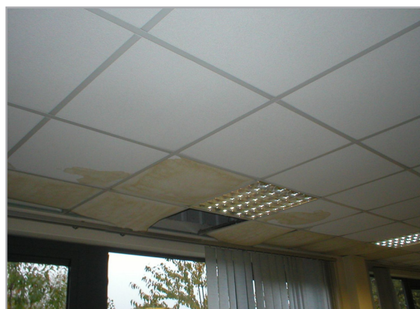
Damage caused by inadequate roof drainage
