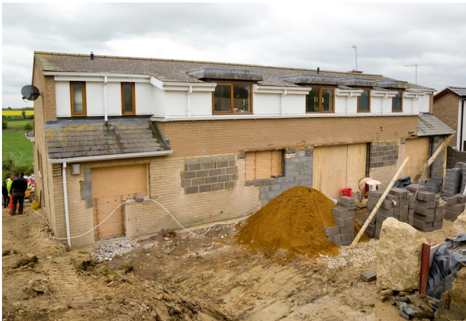
The property during refurbishment
