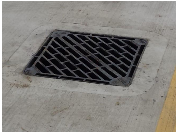
Vented manhole lid for siphonic system
