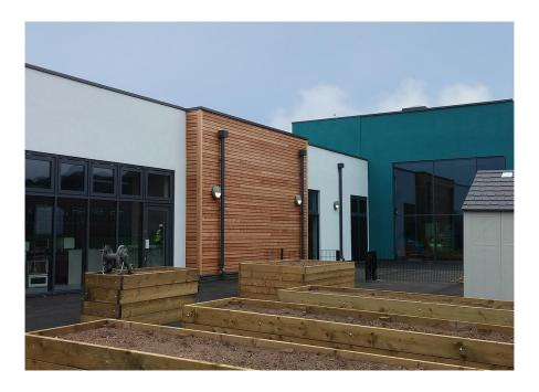
The designs for the Trueline fascia, soffit, wall copings, hoppers and double tiered hoppers were supplied to ARP whose in-house CAD team interpreted the drawings and converted the bespoke designs into CAM drawings for production purposes. All the products were manufactured at its tailor-made manufacturing facility in Leicester and Polyester Powder Coated (PPC) in Slate Grey - RAL 7015 Matt.
