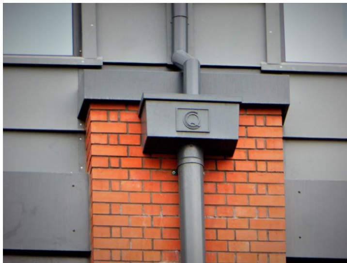
Cast aluminium rainwater hopper Image courtesy of Guttercrest Limited
