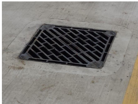
Vented manhole lid for siphonic system
