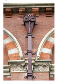
Alumasc worked closely with the main contractors to produce bespoke moulds, creating cast iron replicas of all the existing pipes and hoppers to take away rainwater from the vast single span roof, which is still the largest of its type in the world. Not far away, at the Palace of Westminster Hargreaves Foundry has replaced three large cast iron gutters which after 160 years were being to show signs of wear and tear.
