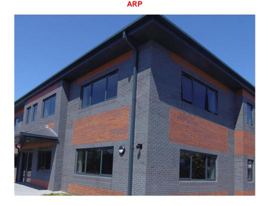
The project was to provide an aluminium rainwater system, including fascias and soffits to a newly built office building in Llanishen, Monmouthshire. The building is likely to be used for offices for multiple businesses as it is ideally situated close to the M4 and Cardiff.
