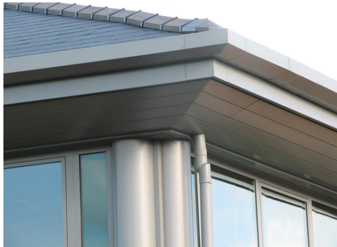
Gutter enclosed by fascia/soffit. Image courtesy of Guttercrest Limited
