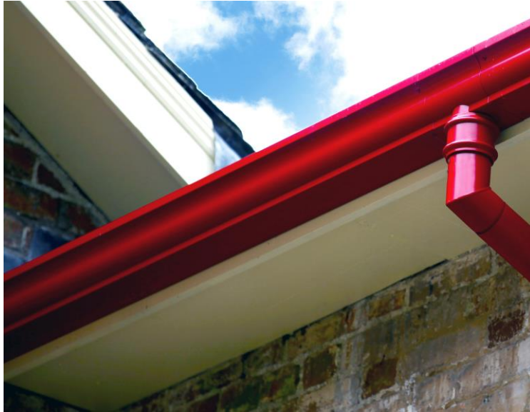
Typical external gutter. Image courtesy of Guttercrest Limited
