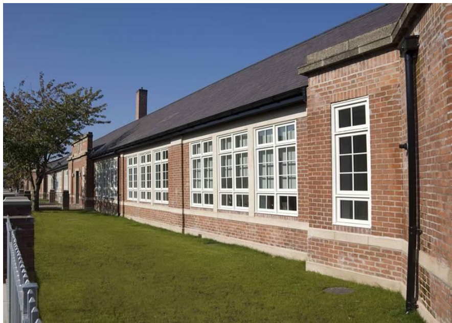
Heritage cast aluminium rainwater system, Mersey Street East Belfast. Image courtesy of Alumasc Exterior Building Products
