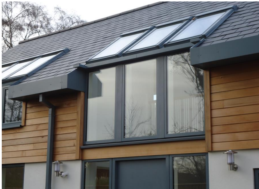
Fascia/soffit system with secret gutter. Image courtesy of ARP Limited
