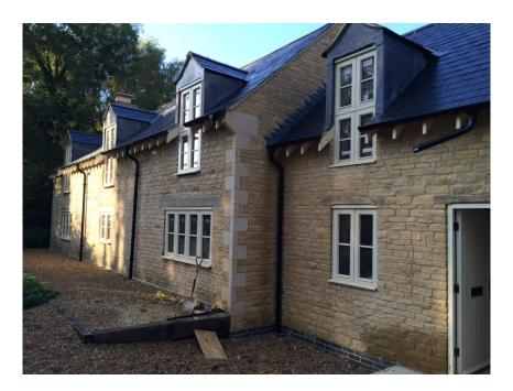
Saint Gobain steel-based Cyclone rainwater drainage system was recently specified for the extension of a listed cottage designed by owner and developer Mark Pollard.
