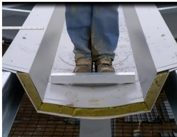
Thin gauge steel and the deflections
