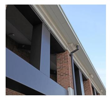
The hotel building, set in landscaped grounds is clad primarily with facing brickwork incorporating contrasting brick coursing and reconstructed stone trims to windows and feature areas. At ground floor level the main public spaces are faced with double glazed aluminium curtain walling to maximise natural light.
