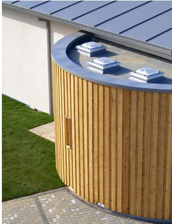
“The roof and gutter design for the new building was a key element in the scheme, as the three mono pitched roofs were designed as a standing seam system, but executed as a single ply membrane with seams. Therefore, we required an elegant and cost effective solution for the very visible roofline.
