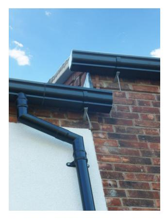
Aluminium is an ideal choice material for the design and manufacture of low maintenance gutters and pipes. It has a high strength to weight ratio and is highly resistant to corrosion. It is a proven material in this application and provides a high level of design flexibility.
