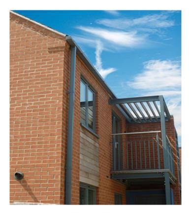
Aluminium is an ideal choice material for the design and manufacture of low maintenance gutters and pipes. It has a high strength to weight ratio and is highly resistant to corrosion. It is a proven material in this application and provides a high level of design flexibility.
