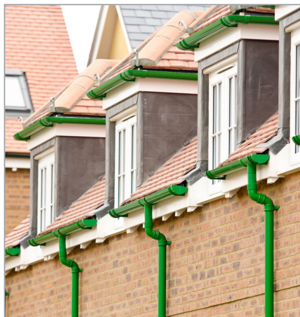
Half round gutter and 63mm Ø downpipe
