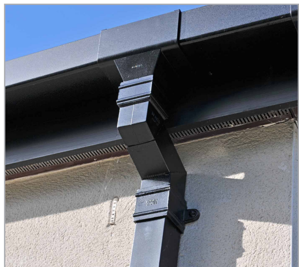
Box gutter and 72x72mm downpipe in textured black finish
